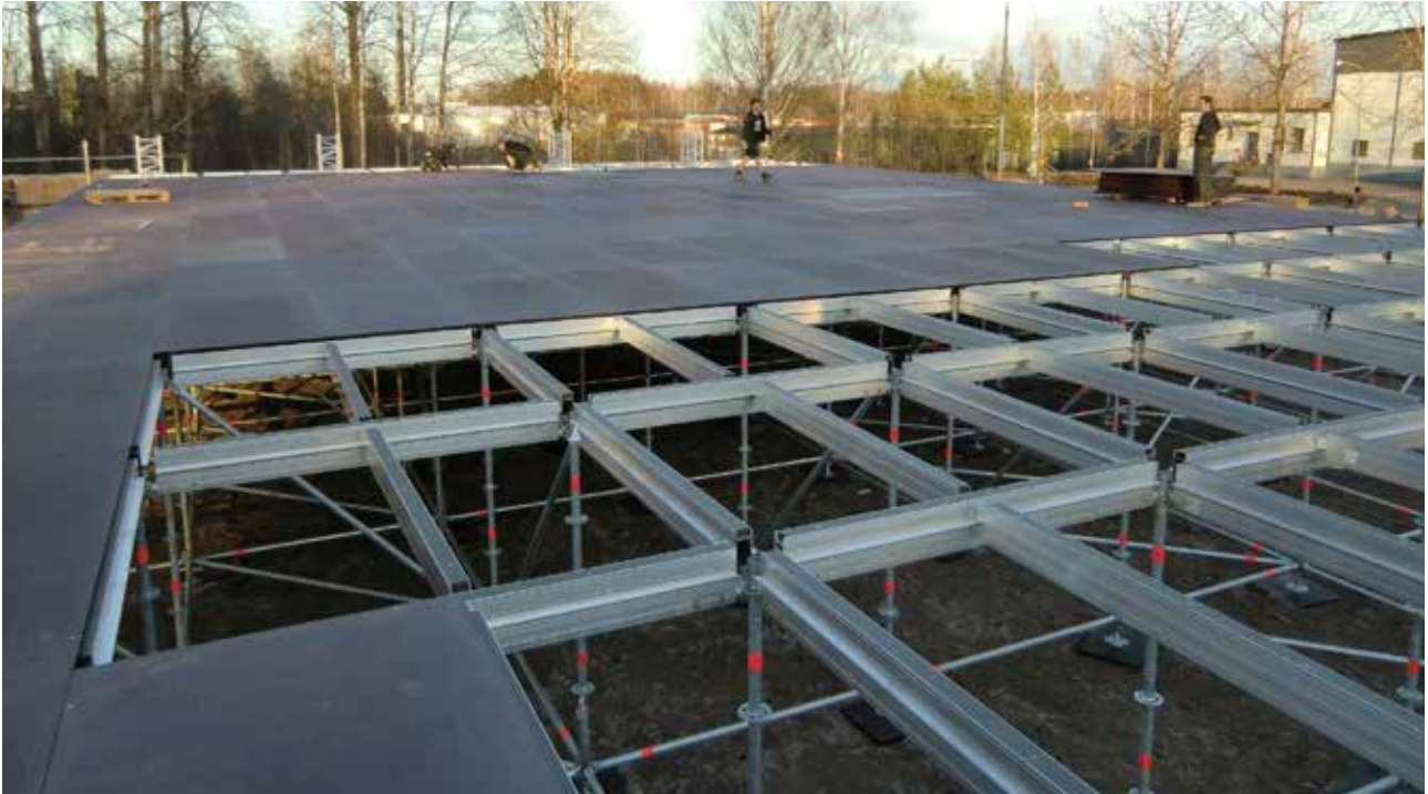
Photo: Prolyte Sales, Space Roof training Starlight
