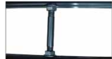
Fig 2. Connection of upper to lower profile by means of stud bolts which are fastened with a self locking nut.
